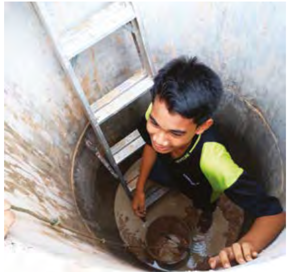
Being courageous while digging the well
